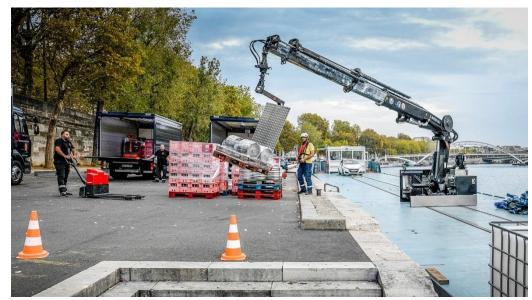
ZULU03's crane in the process of unloading the goods to be placed on to the trucks for the second delivery round. The returnable packaging has been unloaded from the trucks and is waiting to be transferred to the ZULU03, which will then leave on the river for the storage facilities.
